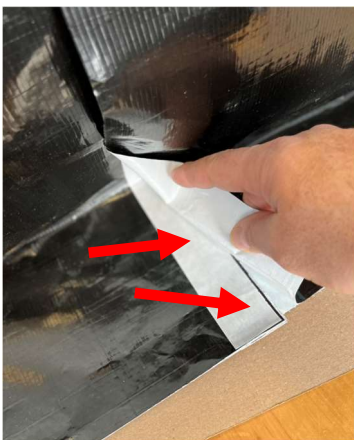
Fig 8 - LOCATE LINER
