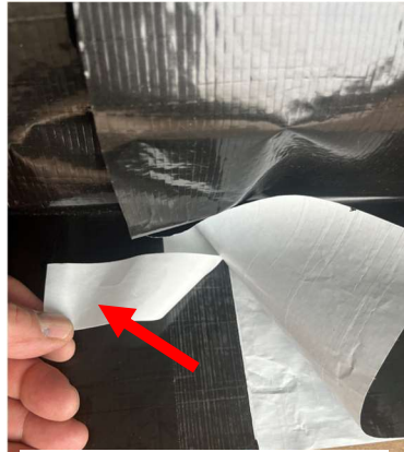
Fig 13 - REMOVER LINER
