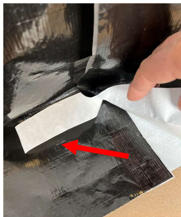
Fig 9 - REMOVE LINER
